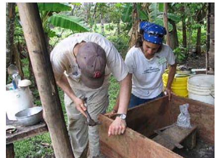
Wood Conserving Stove Construction
