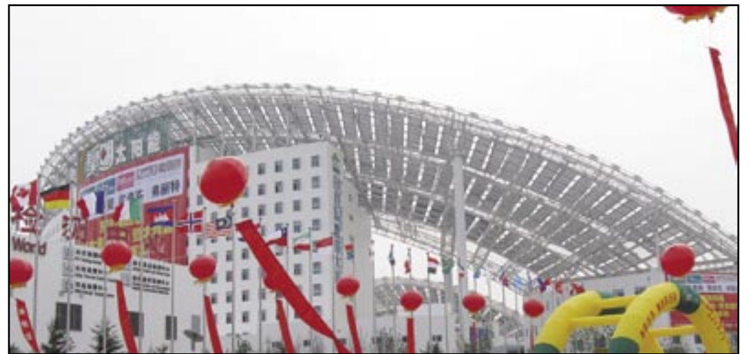
A solar-powered hotel.
